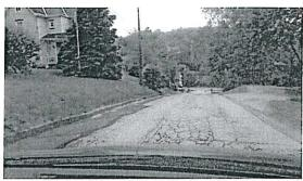
From the data collected, we extract an image that captures every 10-foot 02 section of roadway. These images are analyzed, using machine learning, to identify pavement surface damage such as cracks, potholes, seals, patches, and crocodile cracking. These individual ratings are also aggregated into intersection-to-intersection scores for use in planning.
