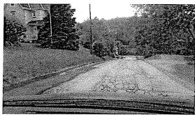
From the data collected, we extract an image that captures every 10-foot section of roadway. These images are analyzed, using machine learning, to identify pavement surface damage such as cracks, potholes, seals, patches, and crocodile cracking. These individual ratings are also aggregated into intersection-to-intersection scores for use in planning.
