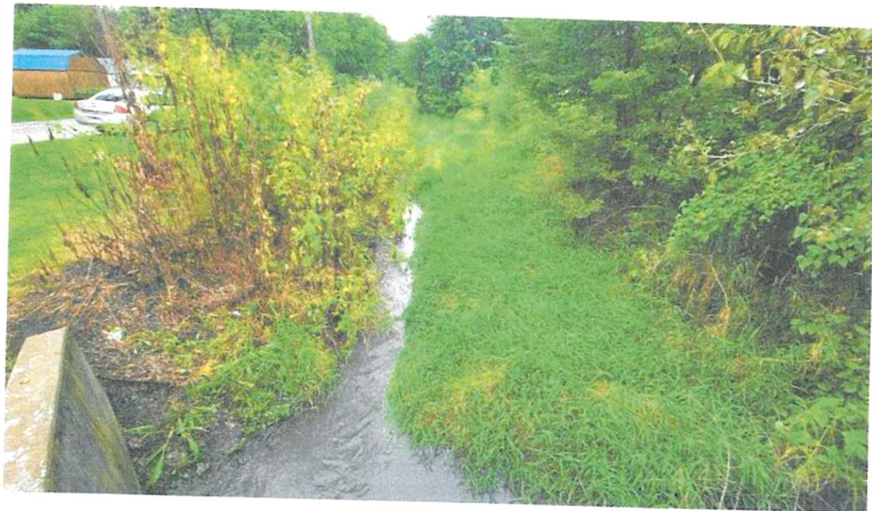
Plum St facing west, flow restriction to the right of water's edge, diverting flow stream into south bank. Broad leaf on south bank allowing highwater to erode the bank.
