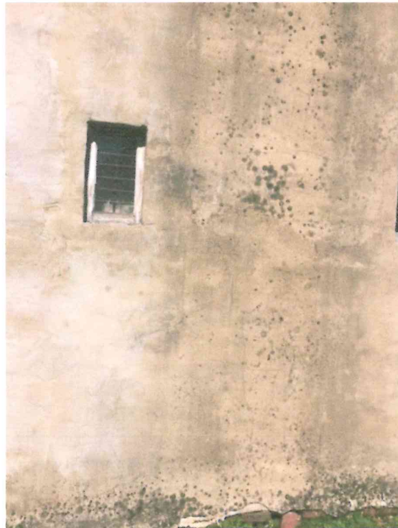
Photograph No. 2 - east elevation close up
