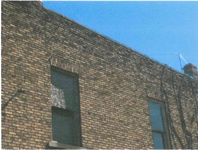
Photograph No. 11 - near the center of the south elevation
