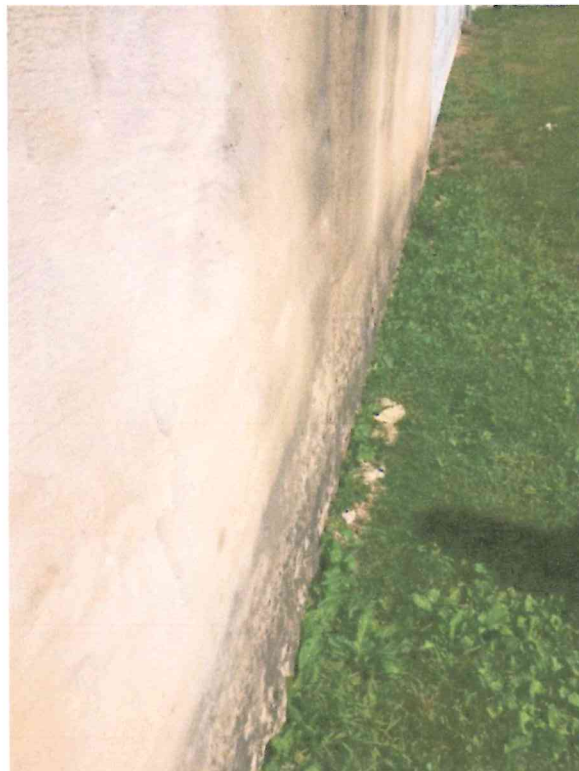
Photograph No. 4 - along east elevation
