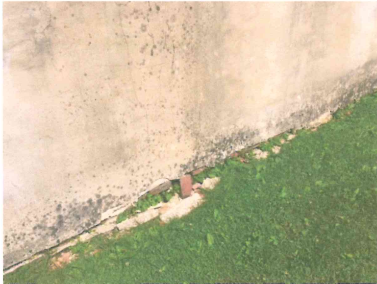
Photograph No. 3 - bottom of wall of east elevation
