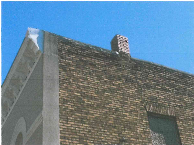
Photograph No. 10 - parapet at west end of south elevation
